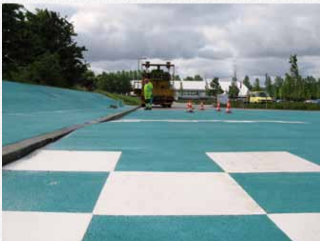
Colourful PREMARK® Anti-Skid in a pedestrian and biking area, where high skid resistance is needed. The applied area is about 1800 m 2 .
