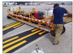
The homogenous composition of AirMark® supports long-term performance regarding bond, retroreflectivity, and UV resistance. The FAA requirements for multi-colored surface signage and delineation markings presents installation and maintenance concerns using traditional application methods. With preformed thermoplastic now included in the AC 150/5370-10F, AirMark® provides a sensible solution with efficient life cycle performance and savings while complementing your total airfield marking program.
